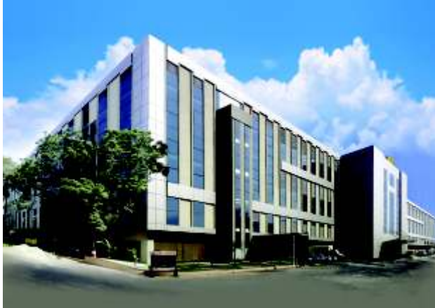
Switchgear Factory, Mumbai
