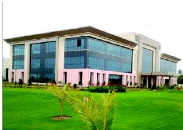
Switchgear Factory, Vadodara
